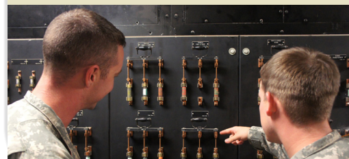
249th Prime Power Unit engineers inspecting critical RCPT facilities
